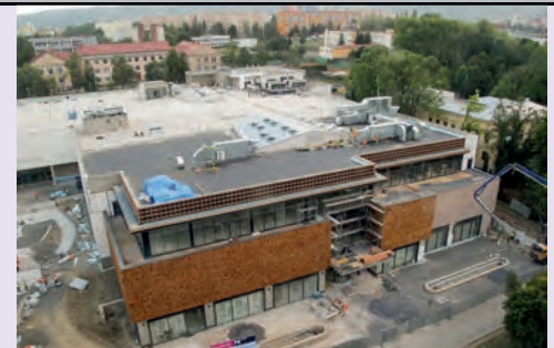
Forum Poprad – construction stage
